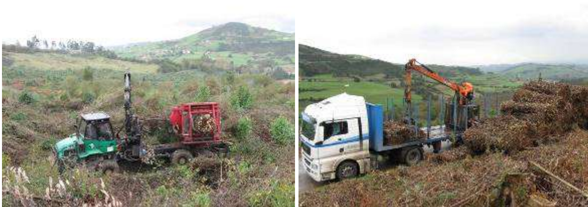
Figure 03-01 18: Baling of loose residues in Northern Spain (left). Bales are then extracted with a forwarder to the roadside where a common timber-truck (right) can autonomously complete the delivery process (source: Gianni Picchi).
