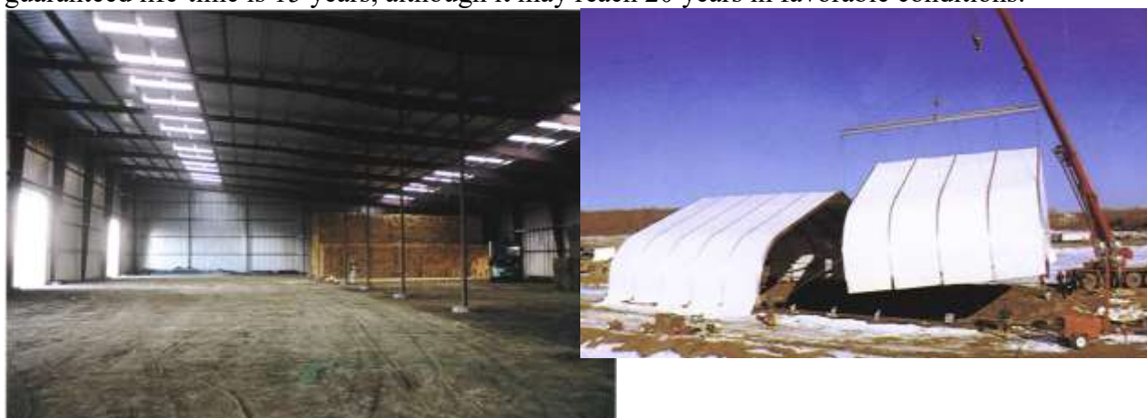
Figure 03-02 7: Interior of metal building for bale storage, left and erection of a fabric building, right (Source: University of California)
