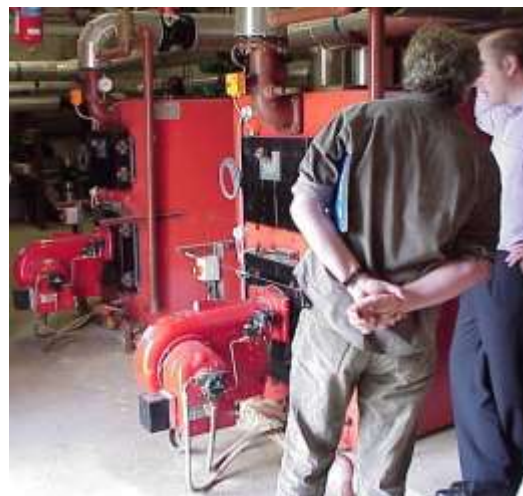
Figure 05-01-03 2: LIT Tipperary, oil tank and oil-fired boiler Photographs by Tipperary Institute
